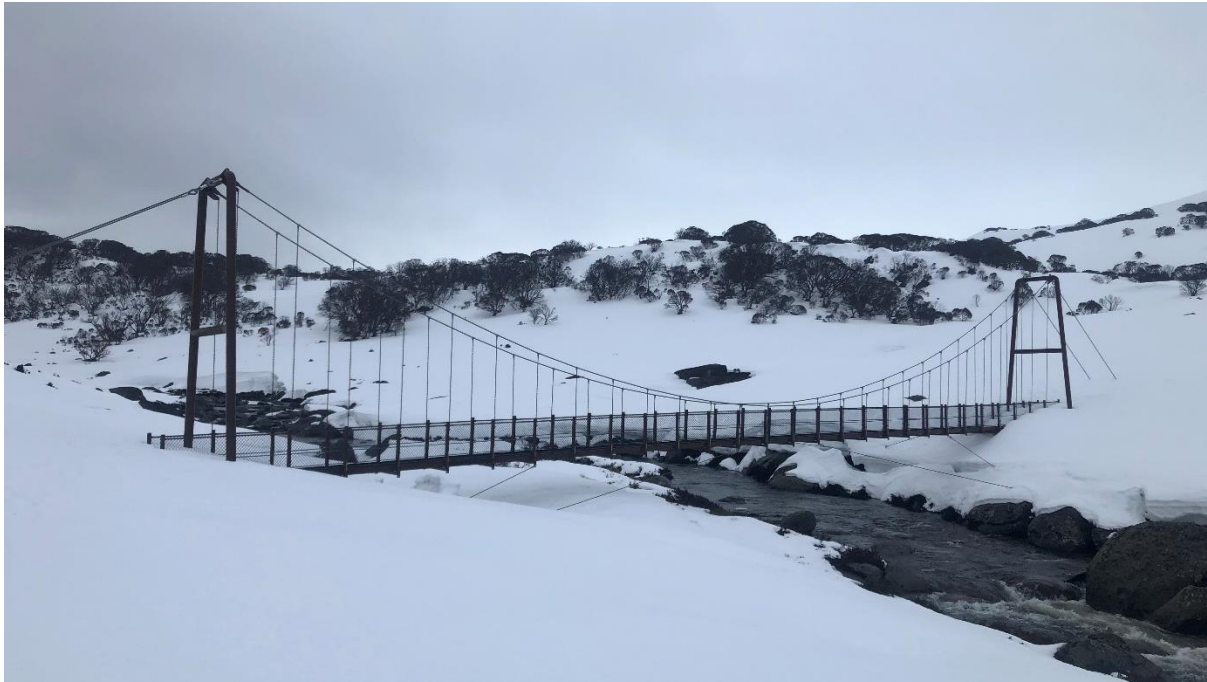
Another record set: the new foot bridge over Spencers Creek is Australia's highest suspension bridge.
