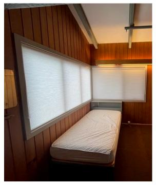
30 double-cell, honeycomb blinds have been installed in the lodge's new windows, here shown in room 5. The blinds are unobtrusive when open and improve insulation when shut.
